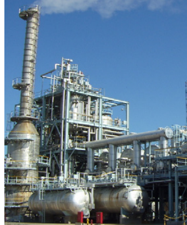
PA Plant at Ulsan Plant
