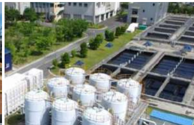
1. Wastewater treatment facility at Ulsan Plant 2. Ulsan Petrochemical Industry Complex Lava discharge water reuse facility
