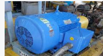
Ulsan Plant P-2 Motor Replaced
