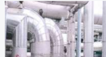
Ulsan Plant P-7 Insulation Reinforced
