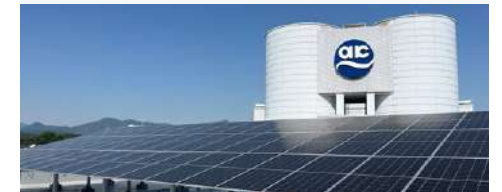
Solar power facility at R&D Center
