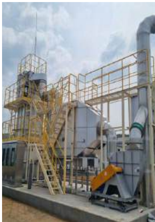
Installation of Odor Control Facilities
