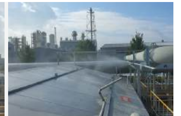
Odor Control System at Ulsan Plant Wastewater Treatment Facility
