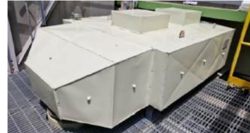
Cheongyang Plant – Economizer Installation
