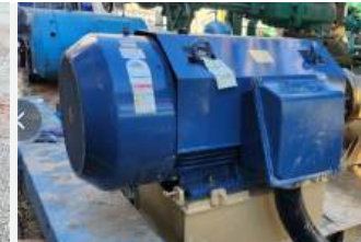
Cheongyang Plant: Replacement of cooling tower motors
