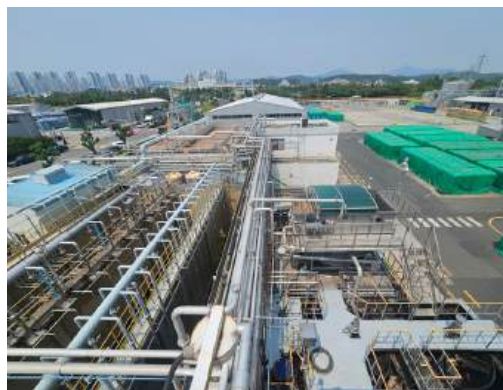
Wastewater Treatment Facility at Ulsan Plant
