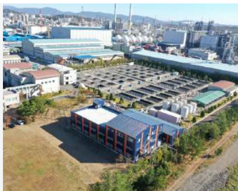
Effluent Reuse Facility at Yongam, Ulsan Petrochemical Complex
