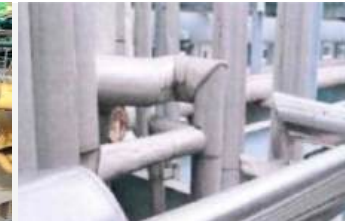
Ulsan Plant (P-5 Plant): Reinforcement of thermal insulation
