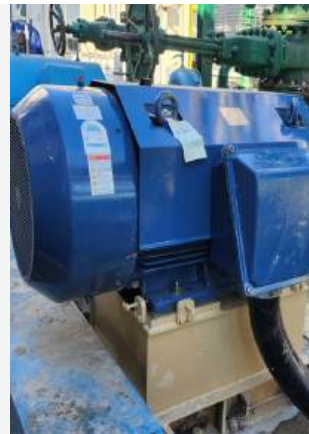
Installation of High-efficiency Equipment
