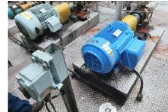
Ulsan Plant: Replacement of motors including G-731A
