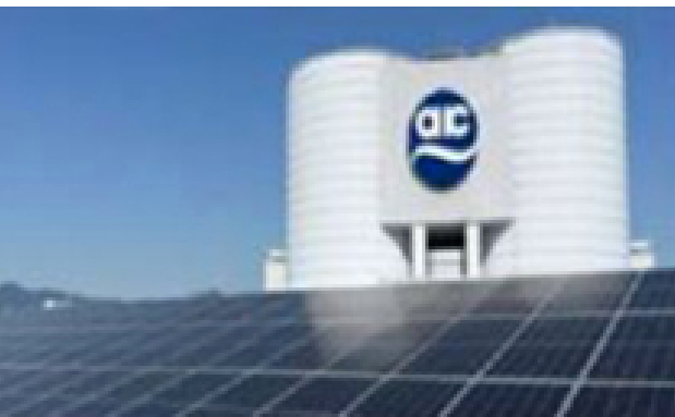
Daejeon Research Center Solar Power Generation Facility
