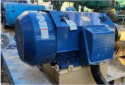
Cheongyang Plant Cooling Tower Motor Replacement
