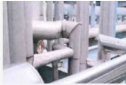
Ulsan Plant P-5 Plant Insulation Material Reinforcement
