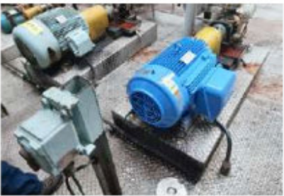
Ulsan Plant G-731A Motor Replacement
